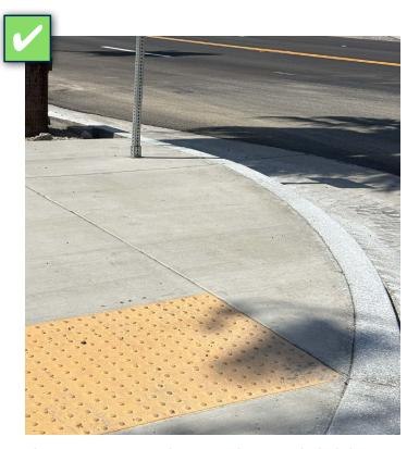
The intersection work at Via Olivera included the install of ADA-accessible ramps.
